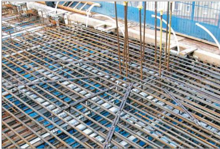
Figure 4 Completed Shearail installation
