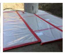
As additional moisture protection a panel section can be put into a foil hose. The endings of the foil hose will be sealed with the repair tape.
