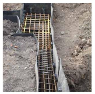
Low strength formwork failing to maintain a neat finished concrete line
