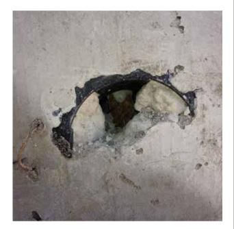
Spacers with small apertures are likely to cause "aggregate lock", preventing adequate compaction and leaving voids around reinforcement bars
