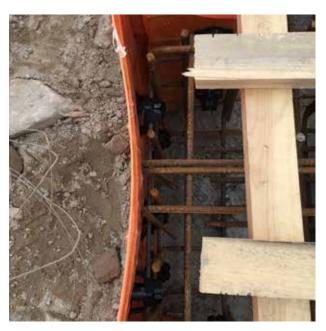
Loss of cover caused by surchage loads from site traffic around excavations
