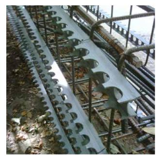
Plastic line spacers were designed for use under fabric reinforcement in flat slabs, not vertical formwork. When turned on their side the concrete is often not able to flow into the channel, creating voids
