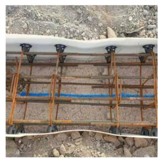
Loss of cover - even with an excessive quantity of spacers - due to inadequate formwork rigidity
