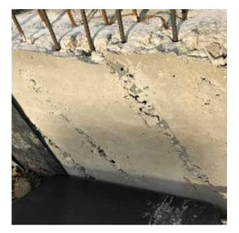
Plastic line spacers are known to cause compaction problems and when used in long lengths may act as a crack inducer
