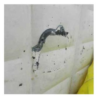
Suitable plastic spacers, like those supplied as part of the Pecafil system, have large apertures to enable coarse aggregate to penetrate and achieve good grout flow
