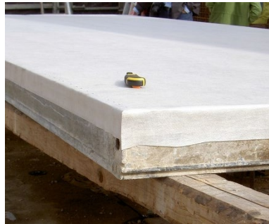
MAX FRANK formwork liner self- adhesive mounted on the formwork
