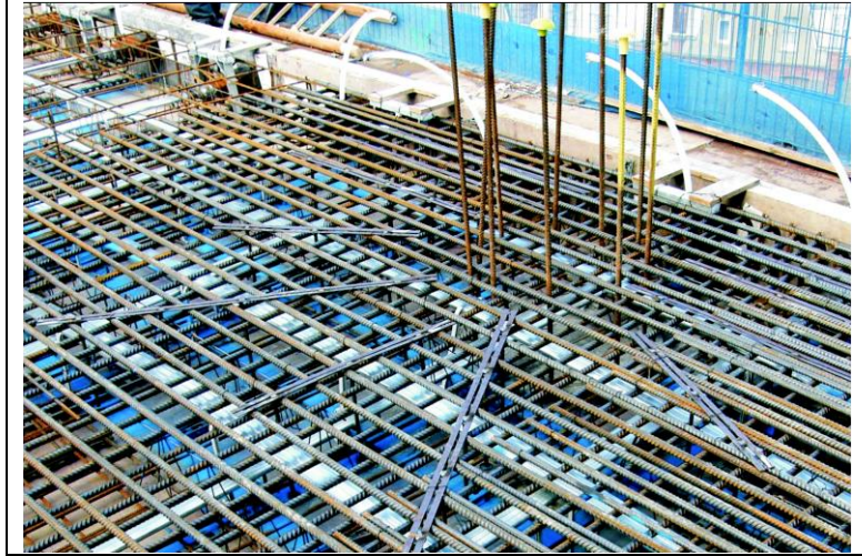
Figure 5 Completed Shearail installation
