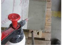
b) Afterwards, the base sealant "Aquafin-IC" from Schomburg was mixed in a small bucket and then applied several millimetres thick over the Zemseal® fleece tape and the concrete surface using a brush to apply.
