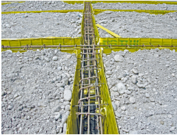
Permanent formwork Pecafil® - foundation formwork
