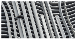
Fibre concrete bar spacers
