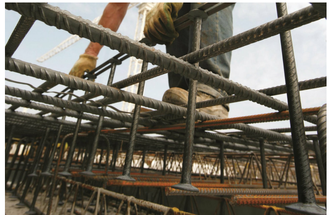
Shearail installation © www.maxfrank.com
