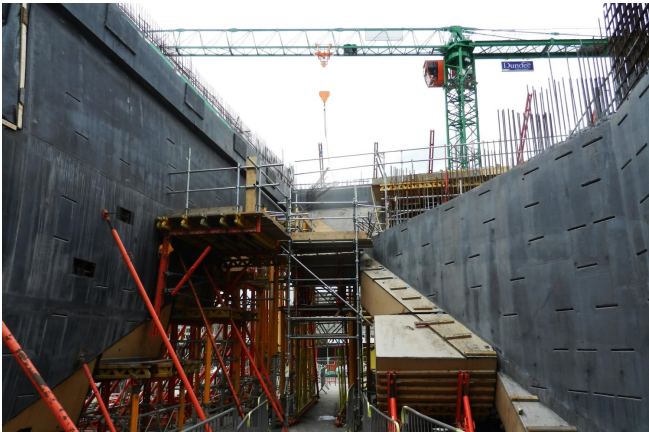
V&A Zemdrain® concrete finish after removal of formwork panels © www.maxfrank.com
