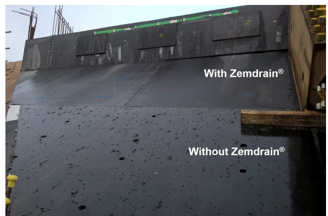
V&A with and without Zemdrain® © www.maxfrank.com
