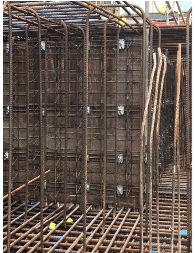
Stremaform® supplied to Anthology Hale Works © www.maxfrank.com
