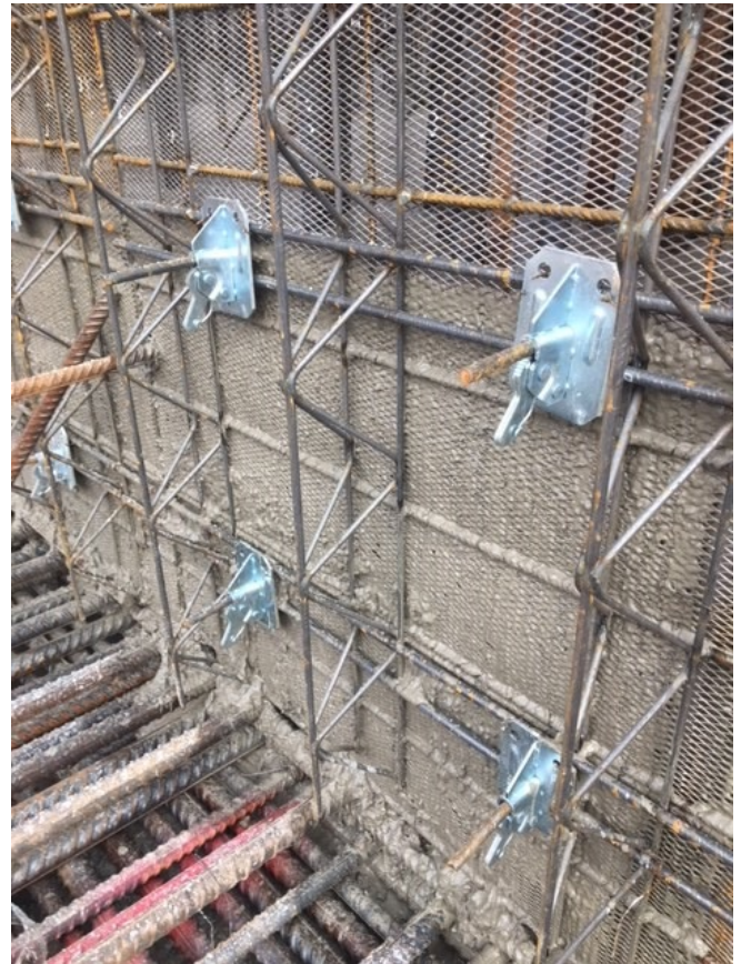
Stremaform® supplied to Anthology Hale Works © www.maxfrank.com
