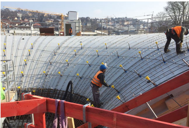
Single spacer on curved component © Bahnprojekt Stuttgart-Ulm, Foto: www.maxfrank.com
