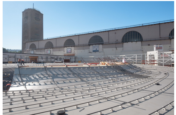
Spacers on formwork for the first chalice-shaped pillar © Bahnprojekt Stuttgart-Ulm, Fotograf: Achim Birnbaum
