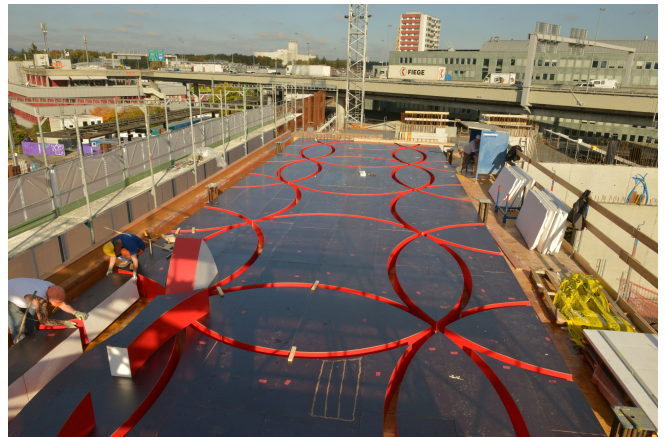
Installation of the shaping formwork Fratec® © www.maxfrank.com
