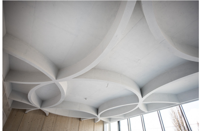
Decorative ceiling realised with shaping formwork Fratec® © Rob Lewis
