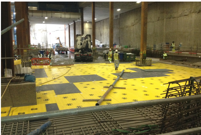
Pecavoid® installation at Heathrow T2B © www.maxfrank.com
