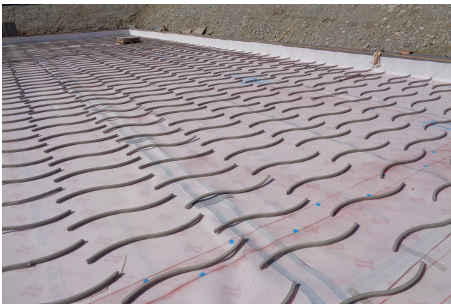
Waterproofing membrane combined with snake type spacers © www.maxfrank.com
