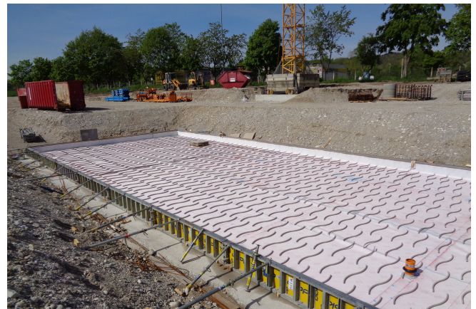
Base plate with waterproofing membrane Zemseal® © www.maxfrank.com
