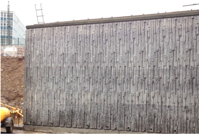
Patterned formwork liners Insitex® Brecon profile © www.maxfrank.com
