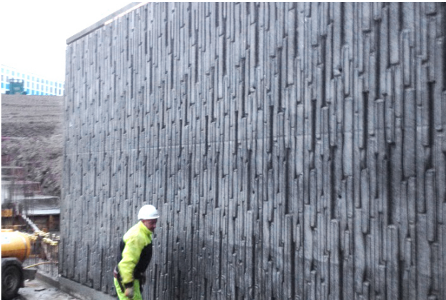
Patterned formwork liners Insitex® Brecon profile © www.maxfrank.com
