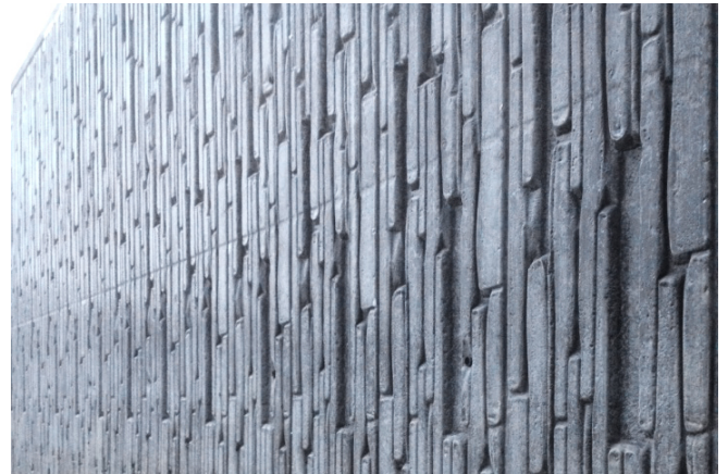
Patterned formwork liners Insitex® Brecon profile © www.maxfrank.com
