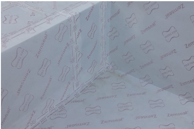
Corner formation with Zemseal® © www.maxfrank.com
