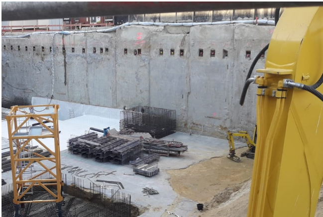
Slotted wall with Zemseal® © www.maxfrank.com
