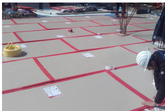
Installation of the Egcovoid® void former © www.maxfrank.com
