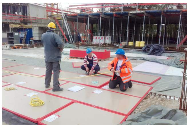
Installation of the Egcovoid® void former © www.maxfrank.com
