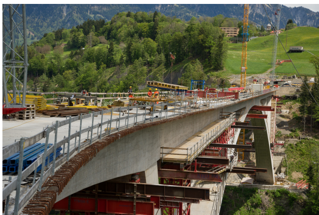
Tamina Valley Bridge © Tiefbauamt Kanton St.Gallen
