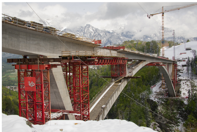
Tamina Valley Bridge © Tiefbauamt Kanton St.Gallen
