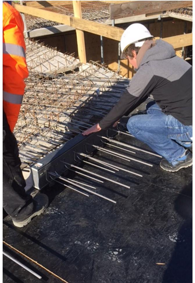
Technical support for the installation of the EgcoBox®
