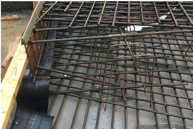
Installation of formwork element Stremaform® © www.maxfrank.com
