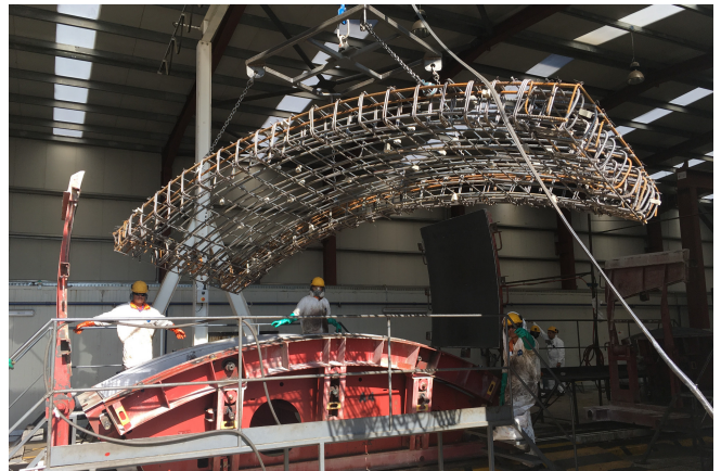
Introduction of reinforcement with fixed spacers into the vibrating formwork © www.maxfrank.com
