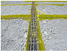
Permanent formwork Pecafil® - foundation formwork
