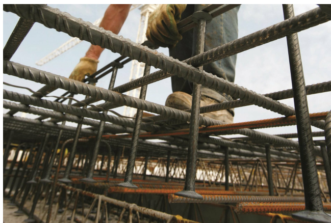
Shearail installation © www.maxfrank.com
