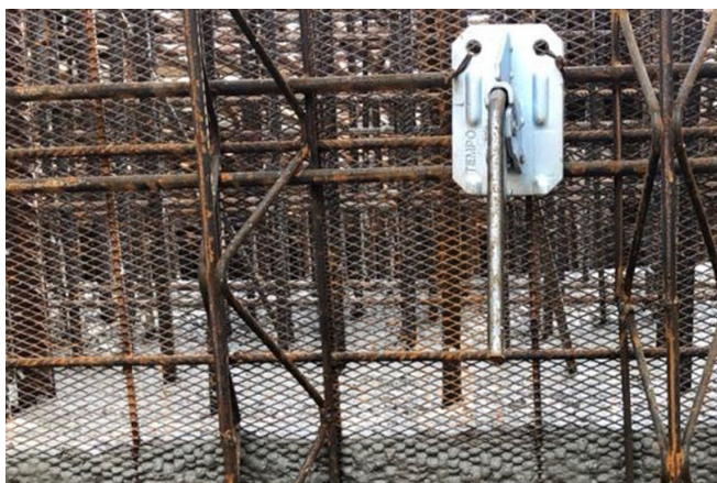
Stremaform® Day Joint Solution © www.maxfrank.com
