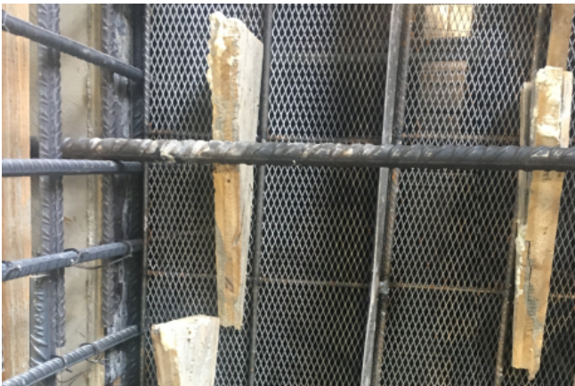
Formwork element Stremaflex® before concreting © www.maxfrank.com
