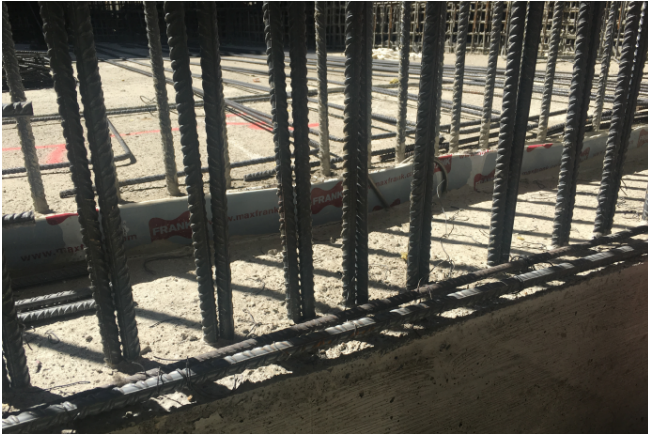
Sealing of the floor slab/wall construction joint with Fradiflex® metal water stop © www.maxfrank.com
