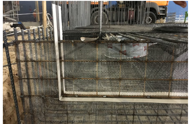
Sealing the floor slabs with Stremaflex® formwork elements © www.maxfrank.com
