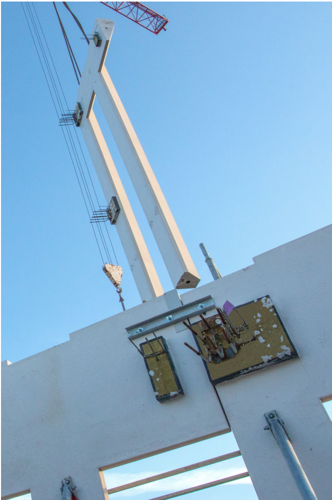
Shear force transmission on the façade element through Egobox® thermal isolating element © www.maxfrank.com
