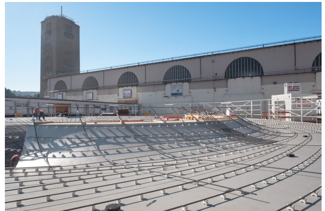
Spacers on formwork for the first chalice-shaped pillar © Bahnprojekt Stuttgart-Ulm, Fotograf: Achim Birnbaum
