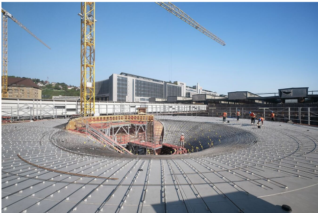
Spacers on formwork for the first chalice-shaped pillar © Bahnprojekt Stuttgart-Ulm, Foto: Achim Birnbaum
