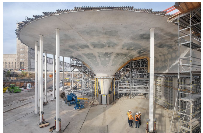
Demoulded chalice-shaped pillar with exposed concrete surface © Bahnprojekt Stuttgart-Ulm, Foto: Achim Birnbaum
