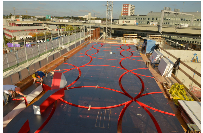
Installation of the shaping formwork Fratec® © www.maxfrank.com
