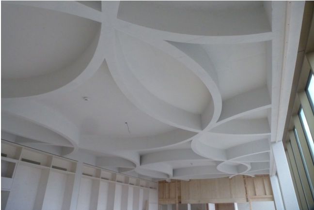
Decorative ceiling realised with shaping formwork Fratec® © Rob Lewis
