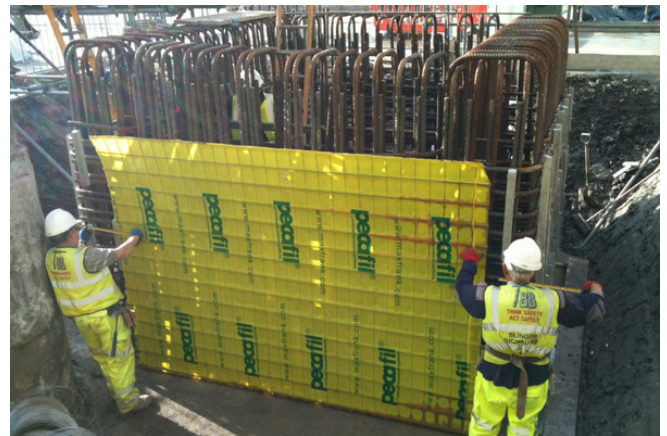
Pecafil® installation at Heathrow T2B © www.maxfrank.com
