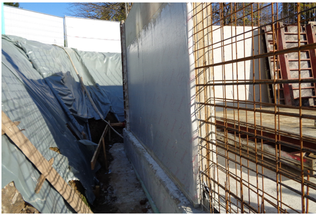
Finished wall surface with Zemseal®. © www.maxfrank.com
