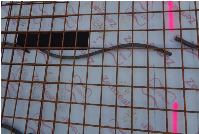
The joints are secured with tape. © www.maxfrank.com
