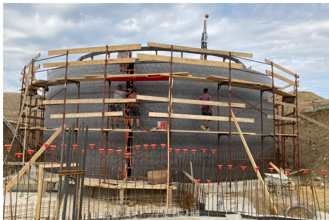
Drinking water tank Henndorf, Zemdrain® CPF liner © www.maxfrank.com
