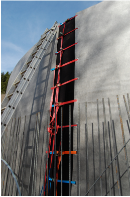
CPF liner Zemdrain® Classic - prefabricated
