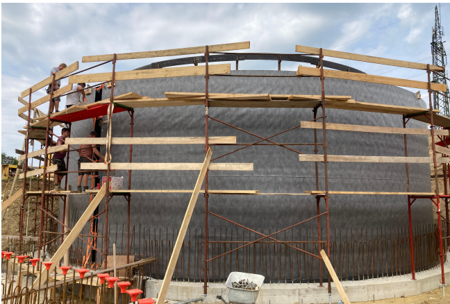
Drinking water tank Henndorfn, Zemdrain® CPF liner © www.maxfrank.com
