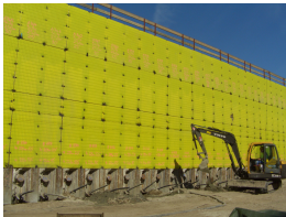
Permanent formwork Pecafil® - foundation separation formwork
