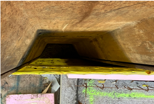
Permanent formwork Pecafil®, foundation separation formwork © www.maxfrank.com
