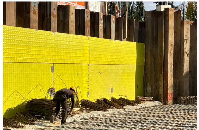
Permanent formwork Pecafil®, foundation separation formwork © www.maxfrank.com
