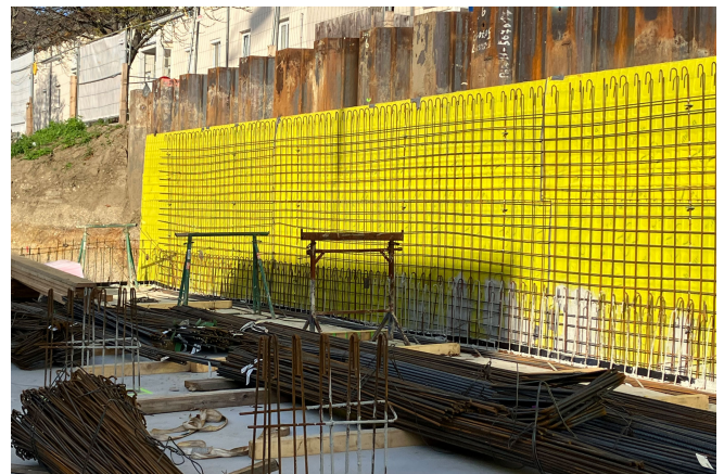
Permanent formwork Pecafil®, foundation separation formwork © www.maxfrank.com
