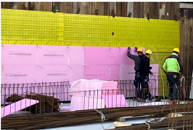
Permanent formwork Pecafil®, foundation separation formwork © www.maxfrank.com
