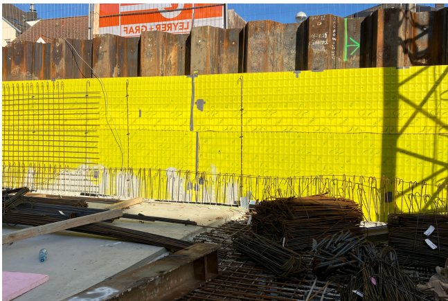
Permanent formwork Pecafil®, foundation separation formwork © www.maxfrank.com
