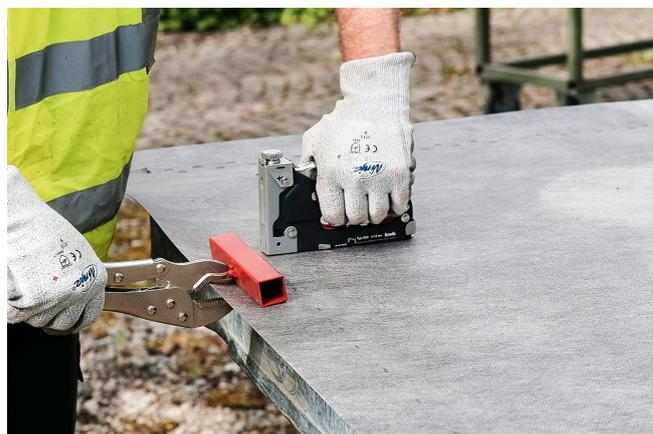
Application example CPF liner Zemdrain® on the formwork
