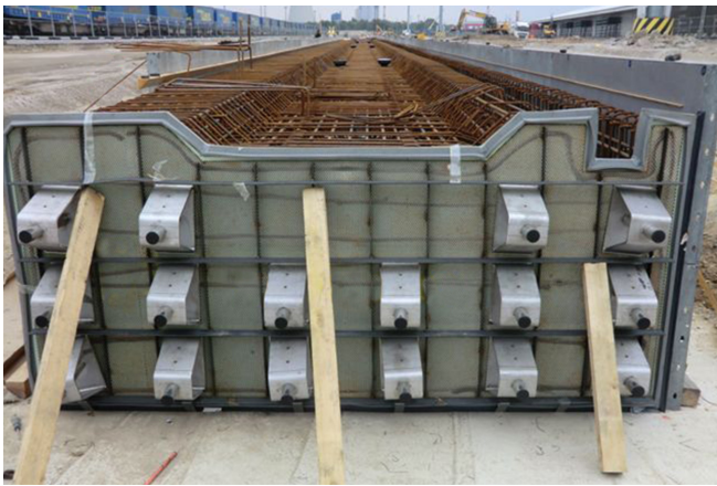
Shear force dowel Egcodorn® for joints subjected to dynamic loads © www.maxfrank.com
