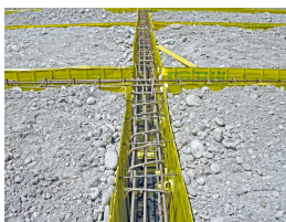
Permanent formwork Pecafile® - foundation formwork
