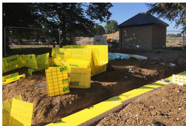
Permanent formwork Pecafile® and ground heave solution Pecavoid® © www.maxfrank.com
