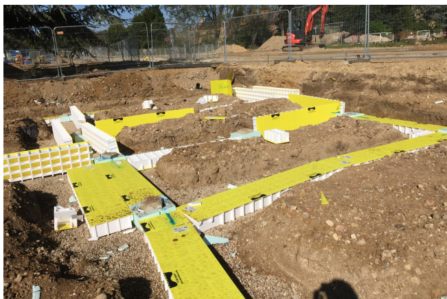
Ground heave solution Pecavoid® © www.maxfrank.com
