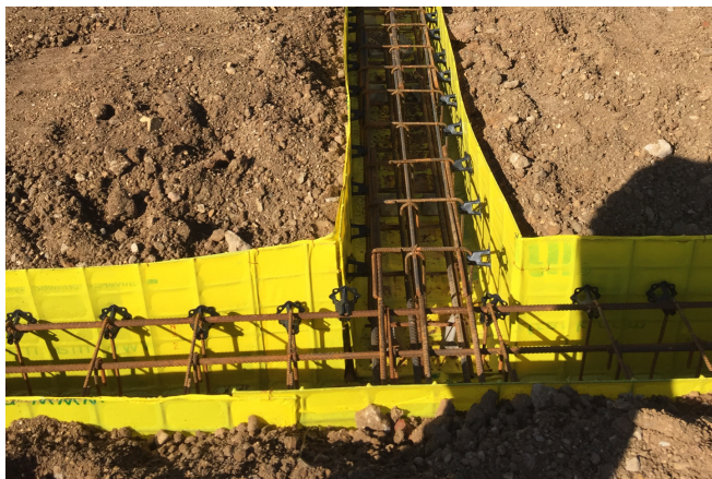
Permanent formwork Pecafile® © www.maxfrank.com
