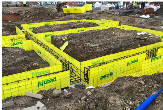
Permanent formwork Pecafile® © www.maxfrank.com
