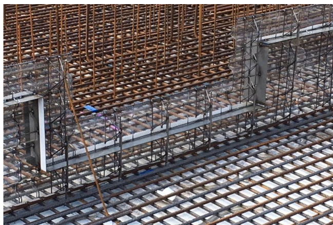
Formwork elements for working joints Stremaform® with coated metall waterstopp © www.maxfrank.com
