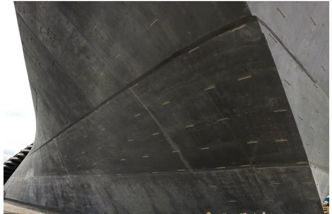
V&A Zemdrain® concrete finish
