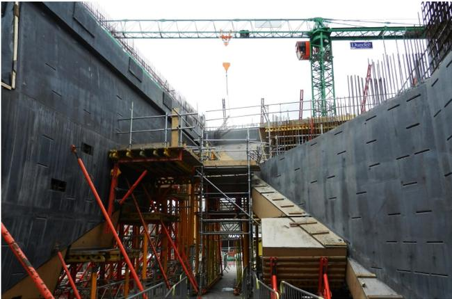
V&A Zemdrain® concrete finish after removal of formwork panels
