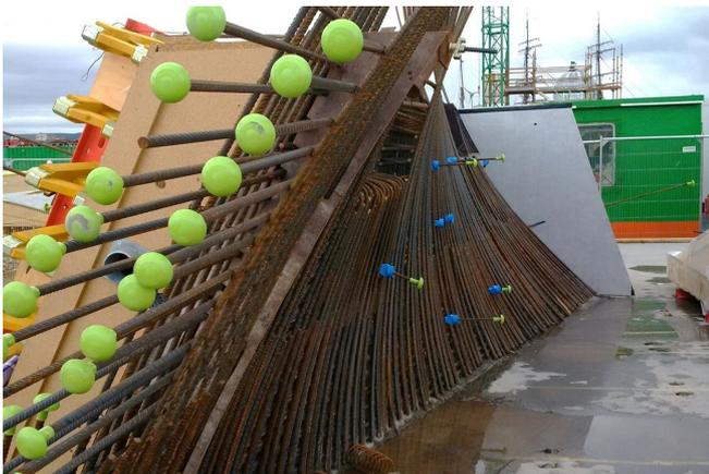
Complexity of structure showing heavy reinforcement cage
