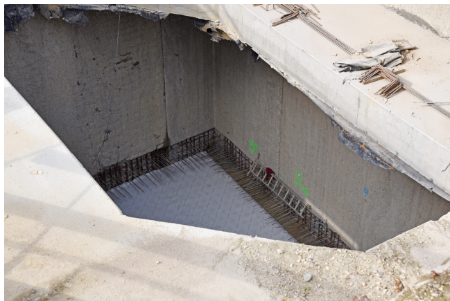
Shaft chamber with laid Zemseal® waterproofing membrane © www.maxfrank.com
