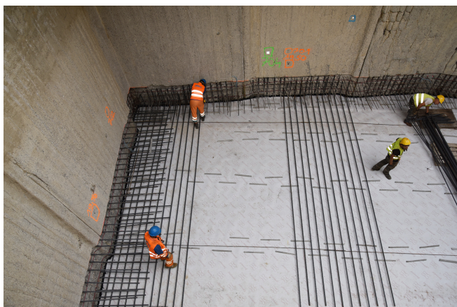
Laying the lower reinforcement layer © www.maxfrank.com
