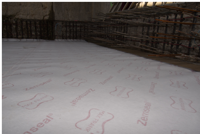
Wrinkle-free layer of Zemseal® sub-structure waterproofing membrane © www.maxfrank.com
