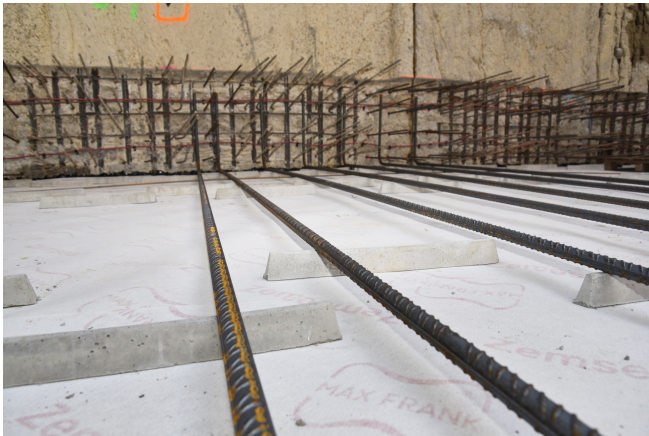
Fibre concrete bar spacer between sub-structure membrane and reinforcement © www.maxfrank.com
