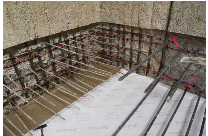
Sealing of the highly reinforced connection area with two grouting circuits of Intec® Premium injection hose © www.maxfrank.com
