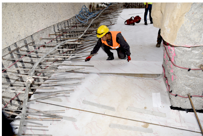
Waterproofing system Zemseal® in combination with Intec® injection hose system © www.maxfrank.com
