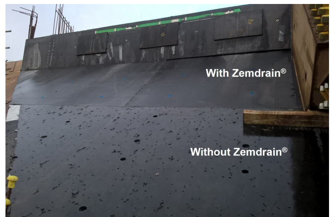
V&A with and without Zemdrain® © www.maxfrank.com
