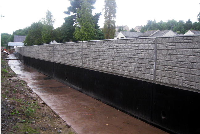
Insitex® patterned formwork liner, Wicklow design © www.maxfrank.com
