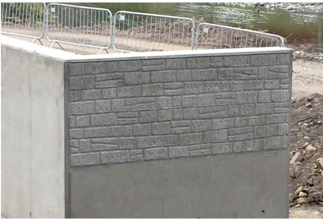
Insitex® patterned formwork liner, Wicklow design © www.maxfrank.com
