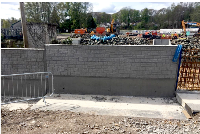
Insitex® patterned formwork liner, Wicklow design © www.maxfrank.com
