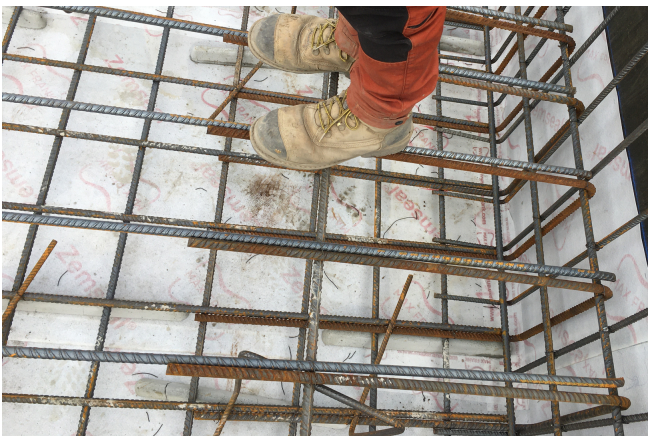
Zemseal® waterproofing membrane installed © www.maxfrank.com
