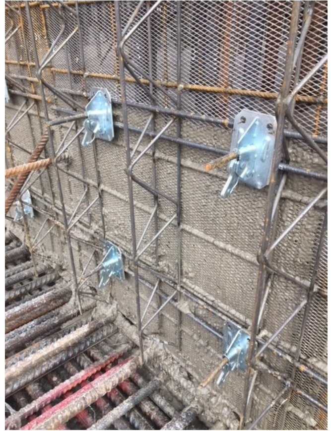
Stremaform® supplied to Anthology Hale Works © www.maxfrank.com
