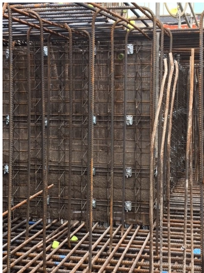
Stremaform® supplied to Anthology Hale Works © www.maxfrank.com
