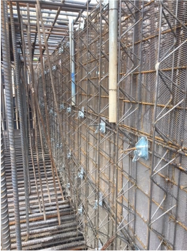
Stremaform® supplied to Anthology Hale Works © www.maxfrank.com
