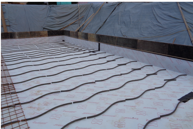
Substructure waterproofing system rolled out © www.maxfrank.com
