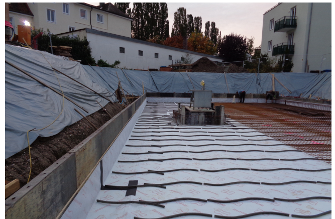
Base plate with lift underpass © www.maxfrank.com
