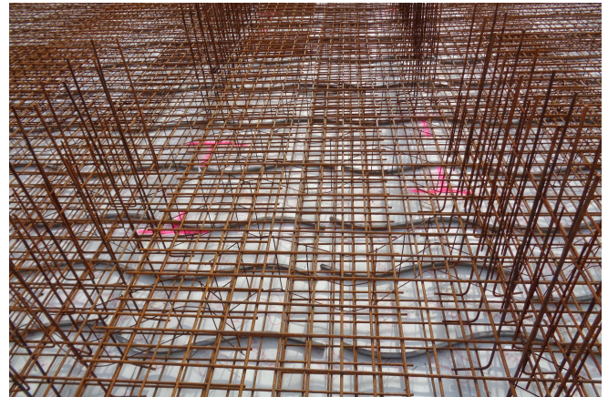
Lower reinforcement layer installed. © www.maxfrank.com
