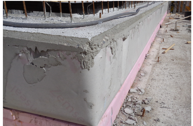
Edge with Zemseal® and Fradiflex® © www.maxfrank.com
