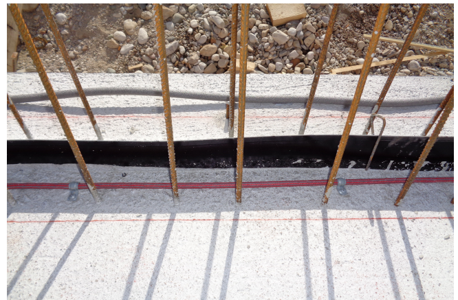
Redundant cold joint waterproofing © www.maxfrank.com
