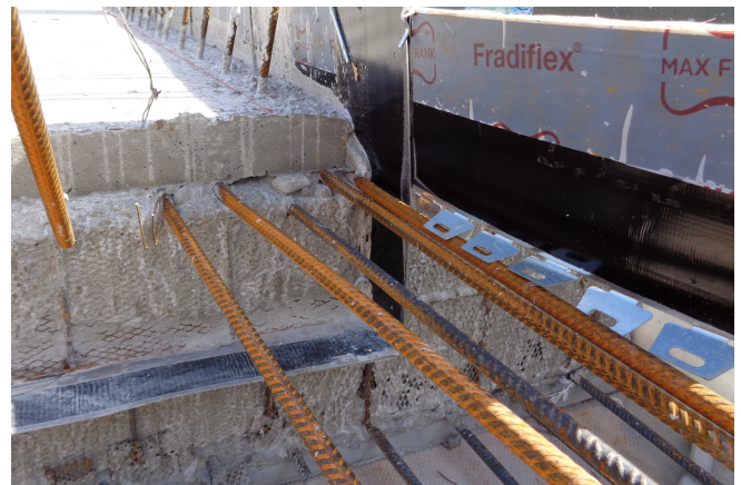
Stremaflex® combined with Fradiflex® with fixing angels © www.maxfrank.com
