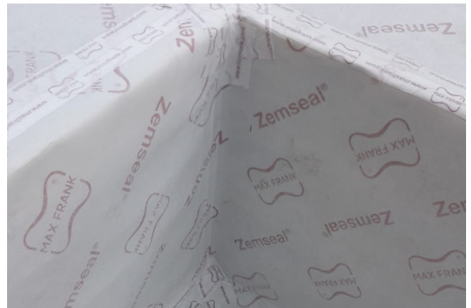
Foundation grounding with Zemseal® © www.maxfrank.com
