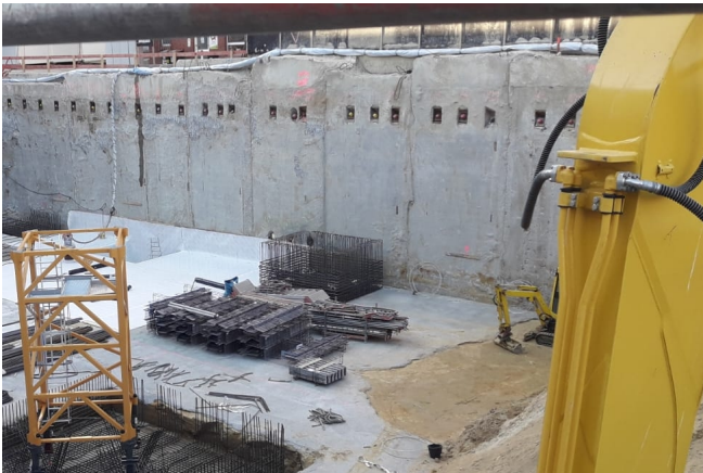
Slotted wall with Zemseal® © www.maxfrank.com
