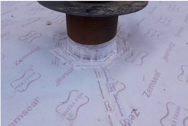
Annular space sealing with Zemseal® © www.maxfrank.com
