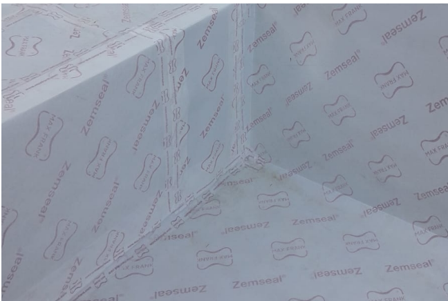
Corner formation with Zemseal® © www.maxfrank.com
