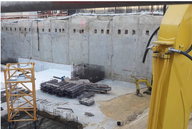
Slotted wall with Zemseal® © www.maxfrank.com
