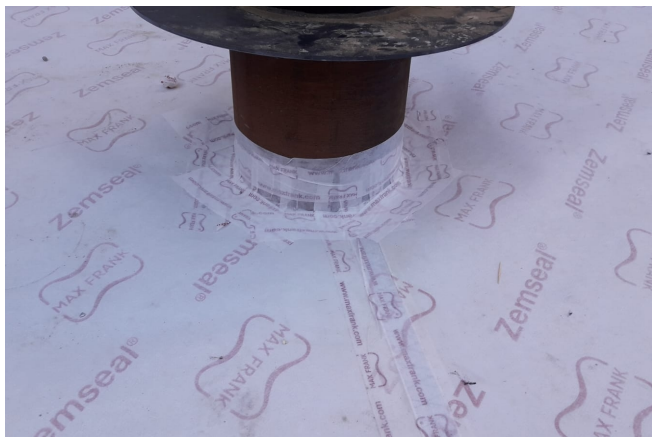
Annular space sealing with Zemseal® © www.maxfrank.com
