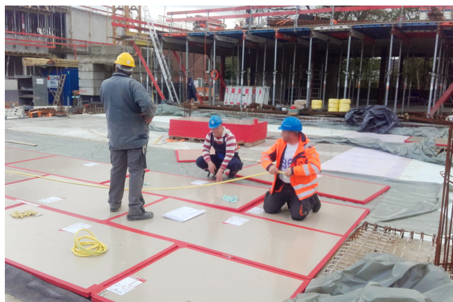
Installation of the Egcovoid® void former © www.maxfrank.com
