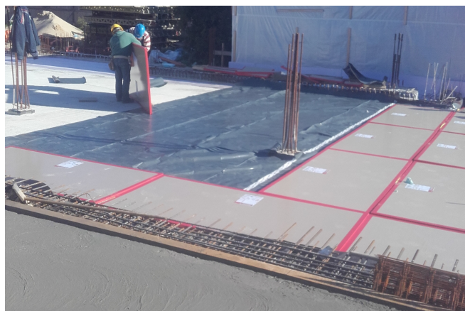
Installation of the Egcovoid® void former © www.maxfrank.com
