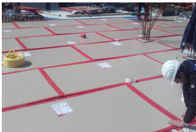
Installation of the Egcovoid® void former © www.maxfrank.com
