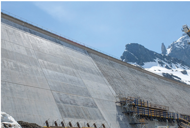
Great Mühldorf Lake dam, with new concrete facing shell under way
