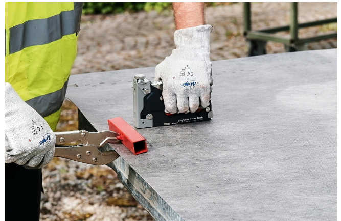
Application example CPF liner Zemdrain® on the formwork
