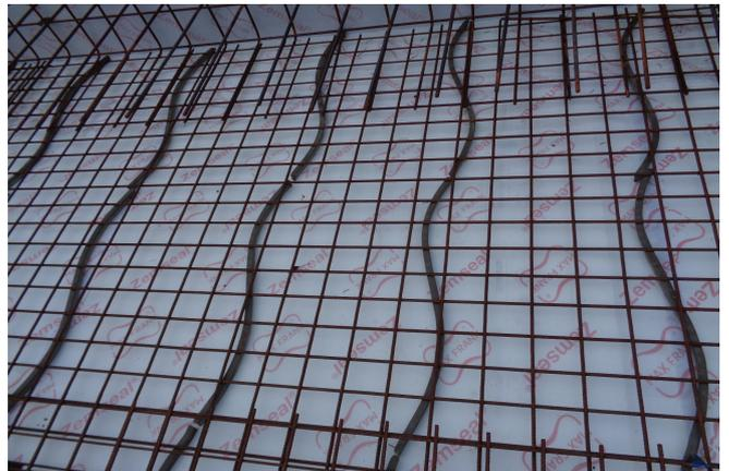
Fibre concrete bar spacers - type snake
