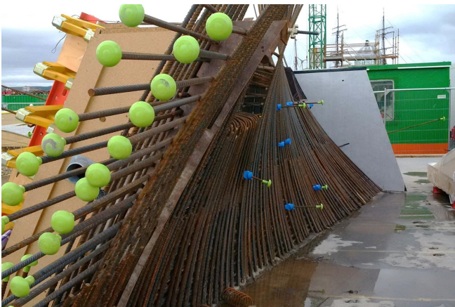
Complexity of structure showing heavy reinforcement cage © www.maxfrank.com
